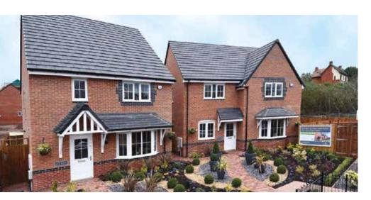
The SIG I-House System can be used where lightweight or traditional construction would be considered and where the design compressive strength of the masonry is approximately  $3N/m^2$ . It is ideally suited for two storey housing and two storeys with room in the roof.
