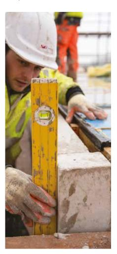
Each unit is constructed by a three man gang and a crane operator from SIG Offsite. This has solved one of the critical challenges faced by Barratt Homes in the Midlands, with a shortage of skilled labour creating a delay in construction. A crane lifts each Celcon Vertical Wall Panel into place where is it secured using a fast-setting mortar specifically created by H+H for use with Vertical Wall Panels.
